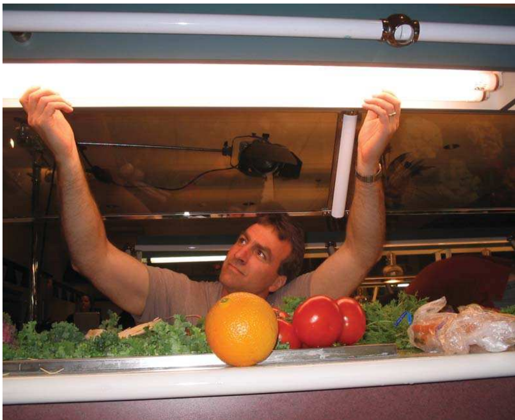
Figure 4.8: Replacing the salad bar lights with Diva Light tubes.
