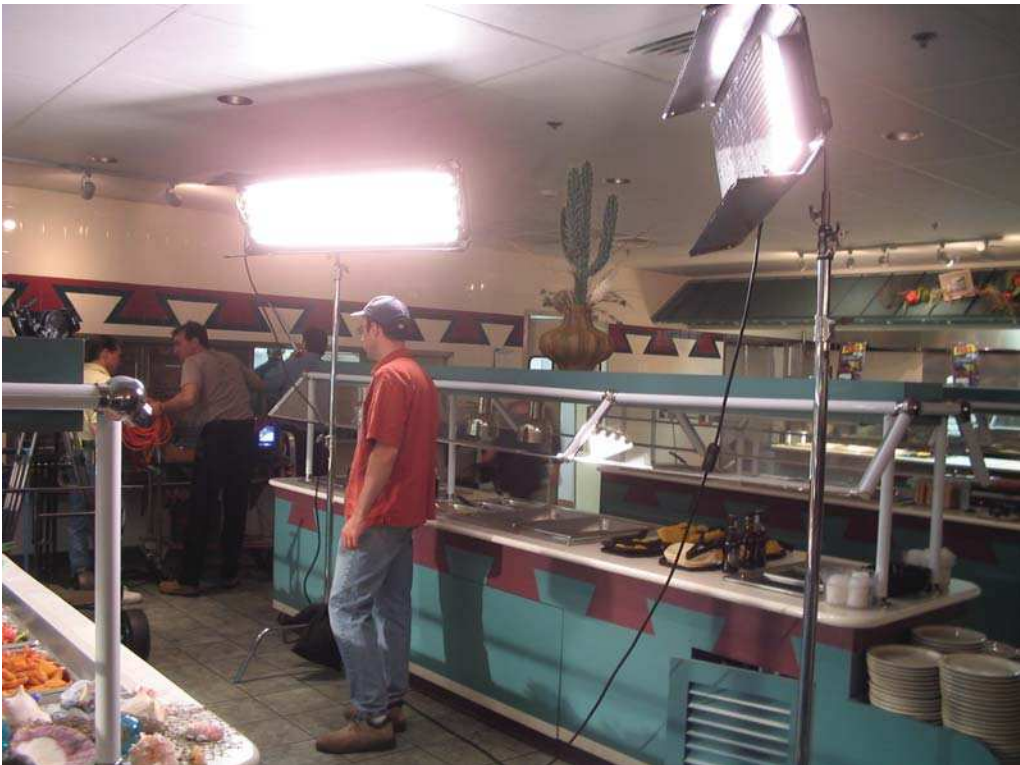
Figure 4.18: Florescent fixtures in a salad bar.
